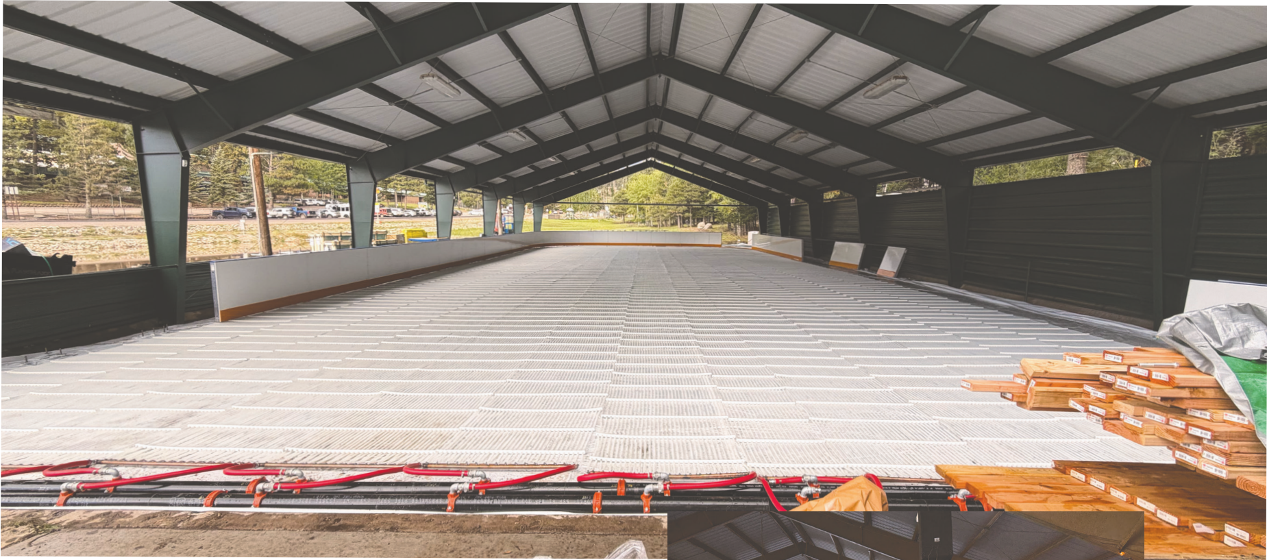
Plans and floor laid: the glycol cooling system is in the rink
