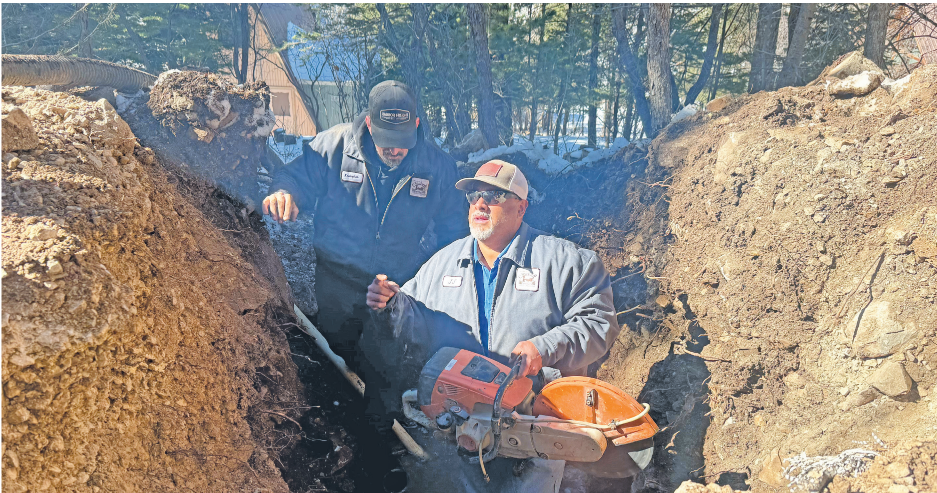
Public Works Supervisor Joe John “JJ” Carrizal and employee Kris Parks install a water pipe isolation valve in the village.
